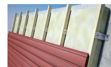
Cladding installation
