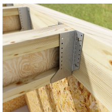
Full nailing on timber
