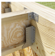
Partial nailing on timber
